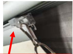
Wand attached to lead panel
